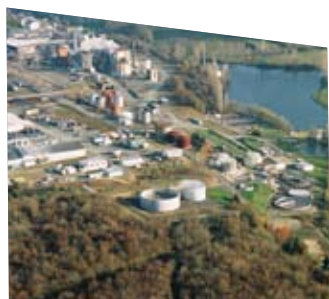
RHODIA OPERATIONS à Melle (79)
